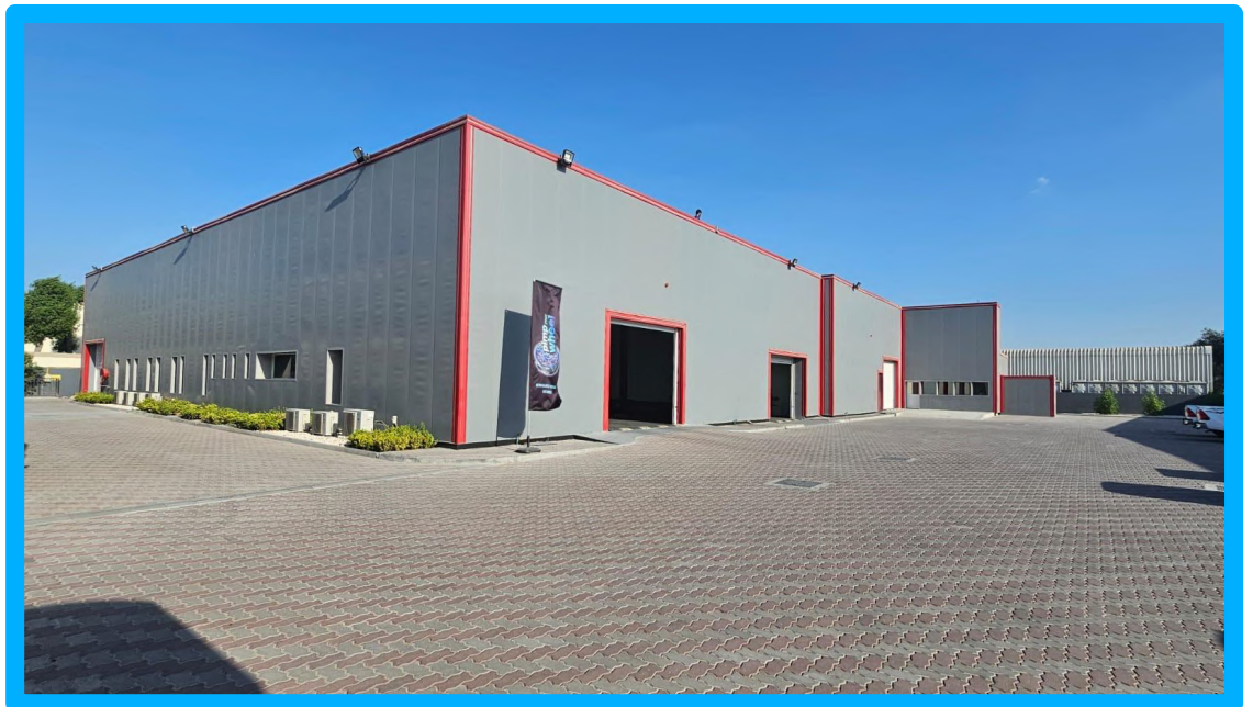
Warehouse Showroom, Al Quoz
